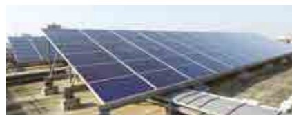
Installation of solar power generation equipment at all facilities
